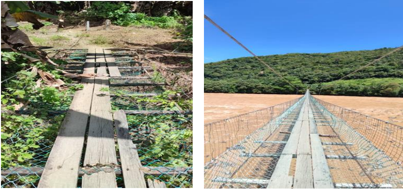
Figure 8 Hanging Bridge Kampung Panggi
