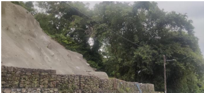
Figure 22 Another look the reinforcement
