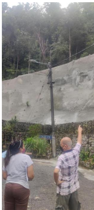
Figure 21 Concrete reinforcement by DBKL to mitigate landslides at Lot 40872
